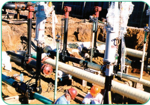
Figure 11 – Installation of Becker Below Ground Regulators (Prior to Backfill)
