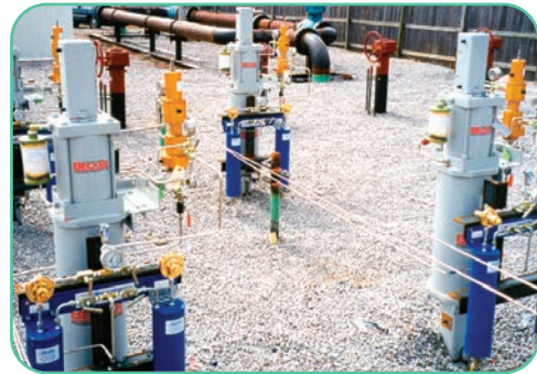
Figure 12 – Installation of Becker Below Ground Regulators (After Backfill)
